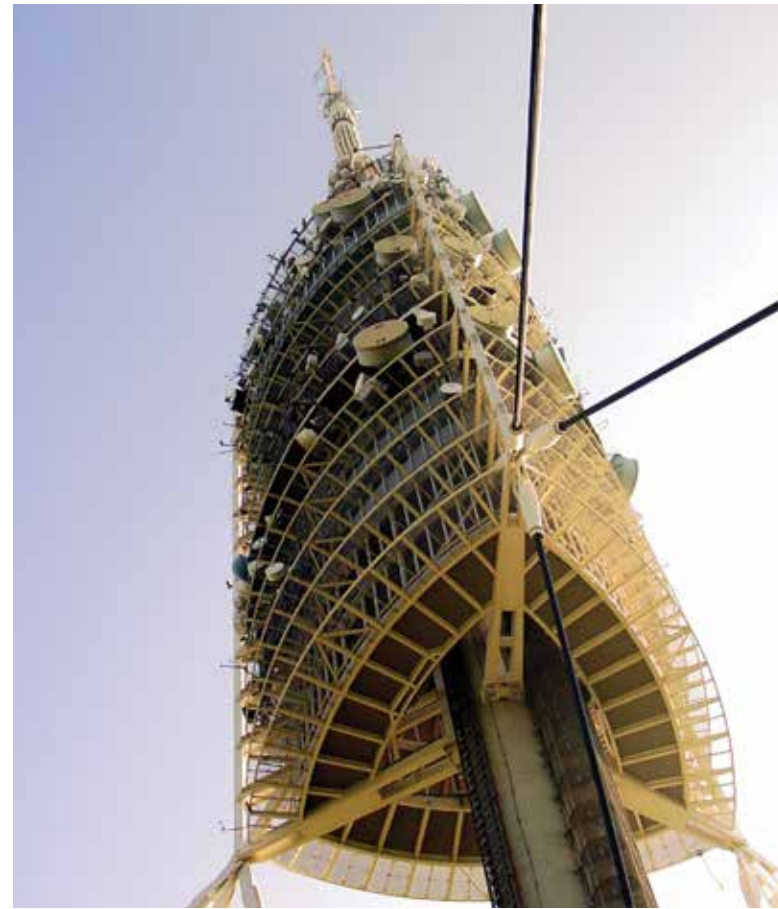
Collserola communications tower, Barcelona
